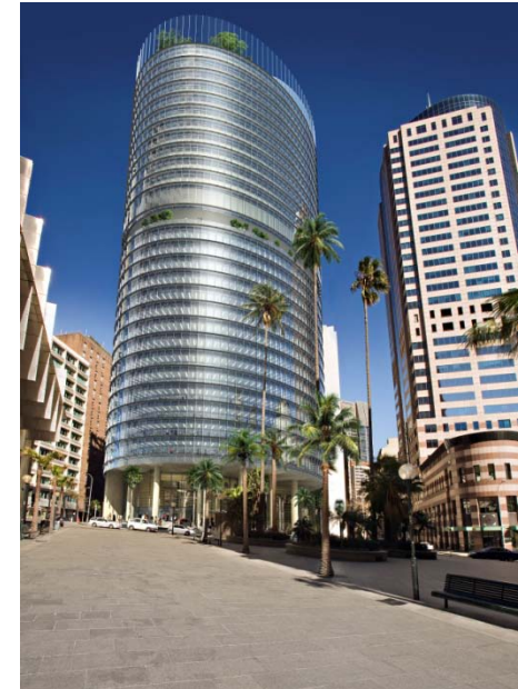
1 Bligh St: 6 green star design, under construction, Sydney CBD
